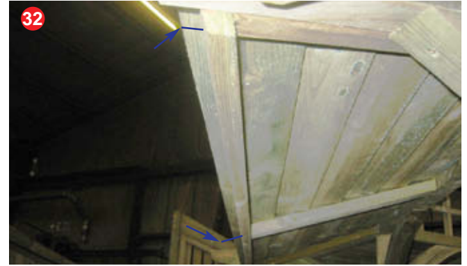
Underneath view of roof coverstrip attachment.
