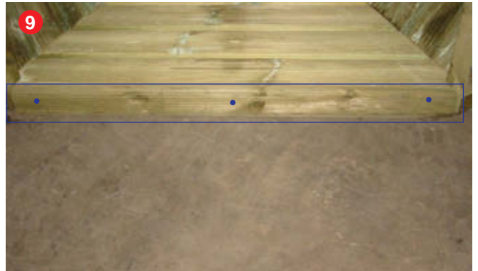
Attach floor edge panels using 3 x 40mm screws
