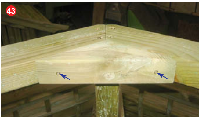
Using 2 x 40mm screws, secure a corner support in each corner of the top frame.
