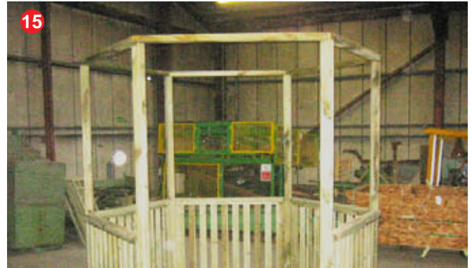
15 Upright top frames are positioned as shown.
