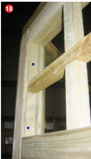
18 Secure fence with 4 x 50mm screws, 2 at each end of the fence.
