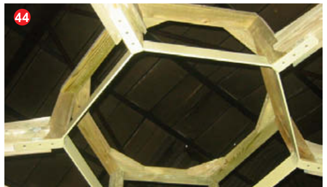
Shows top frames with corner supports in position.
