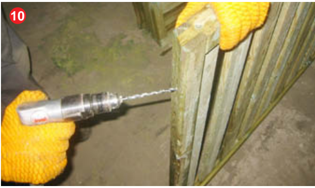
10 Sit the large fence on the floor between the uprights and secure with 6 x 70mm screws. It may help to drill pilot holes in the end frames of all the fence.
