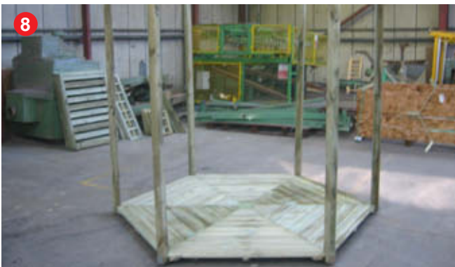
All uprights secured in place.
