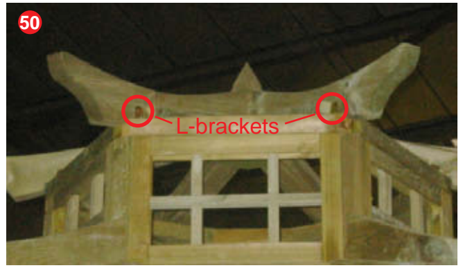
50 Secure top roof bearers to top frame using 2 L-brackets and 8 x 40mm screws per bearer.
