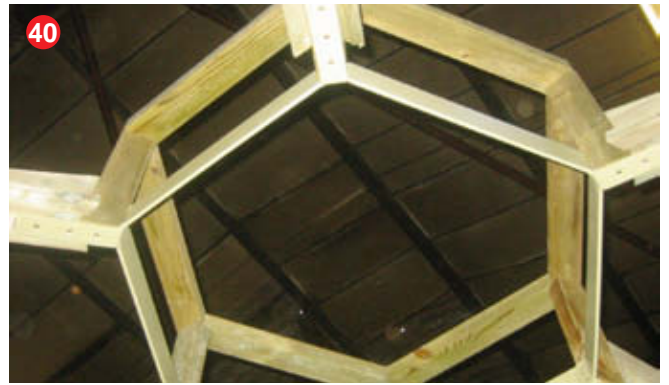
Shows top frames in position.
