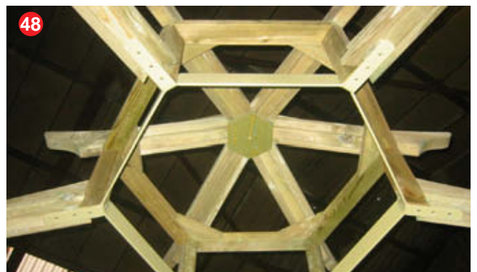
Position bearer assembly centrally onto the top roof frames.
