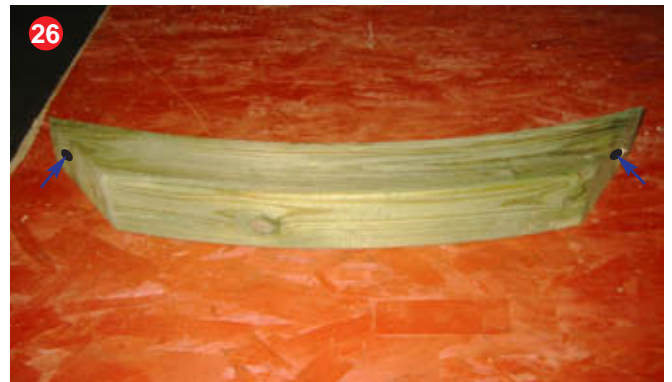
26 Drill a hole in each end of the lower roof bearer support
