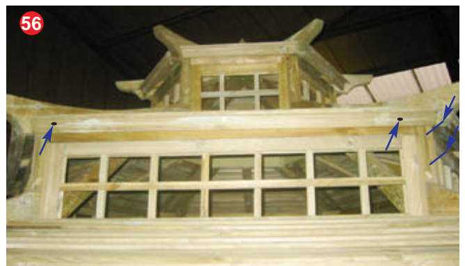
56 Fit 6 roof panel fascia boards and the 6 finials using 2 x 50mm screws each.
