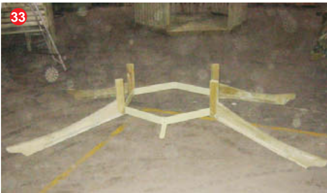
Attach 4 long roof bearers to the metal ring. See 34
