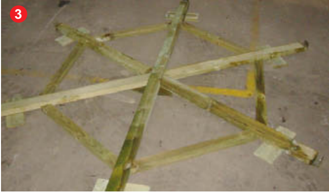
Add floor bearer separators.
